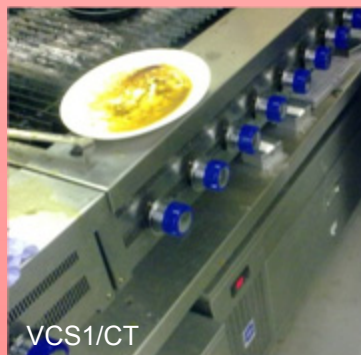
Side Engine Adande Drawer, under Charbroiler, with required air gap above the cover top
